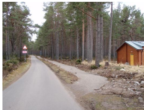
Fig. 5 : end of walkway at Centre
